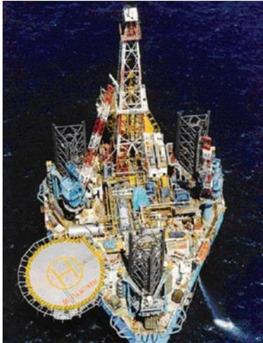
A comprehensive 16,000 BPD Early Production Process System installed onto the Ampolex jack-up rig 'Hakuryu VII' in Dampier, Western Australia, in late 1993. This system was later modified to process up to 28,000 BFPD. The facilities were initially installed to complete a 120 day EWT phase followed by EPF operations if proved commercial.
